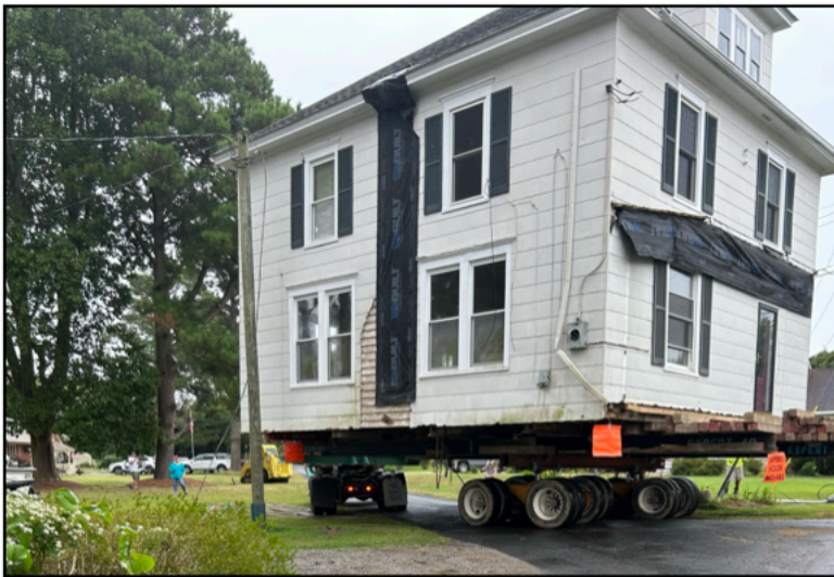
Above, the house came very close to a couple poles and a few trees. Above, right, an 18-wheeler cab pulled in the front, while big dollies rolled in the back. Right, the house sitting in its new location.
