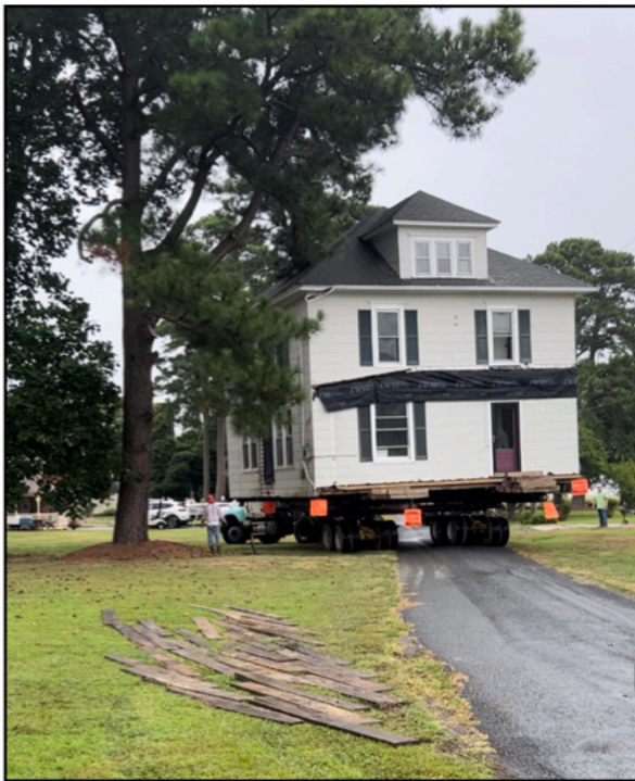
Right, the house makes the final turn into its new space.
