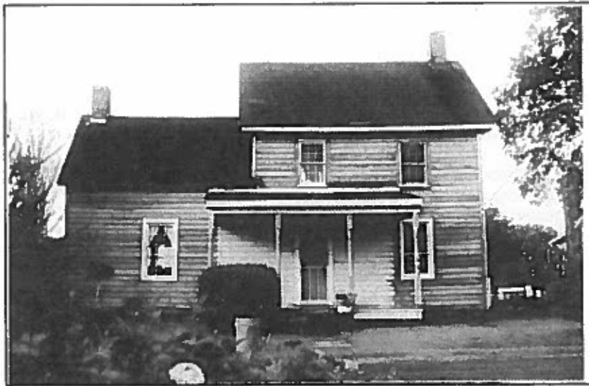
2 South Street, probably built as a "model" house soon after Powellton was founded.
